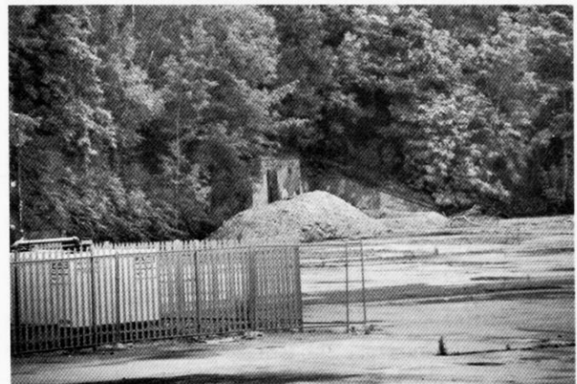
East works tunnel entrance. Photo by Neil Wedgbury.
